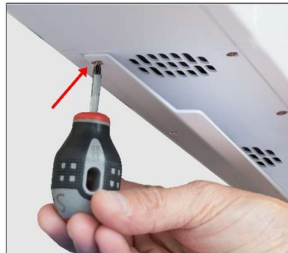
Figure 10 - Sound Deflector Installation
