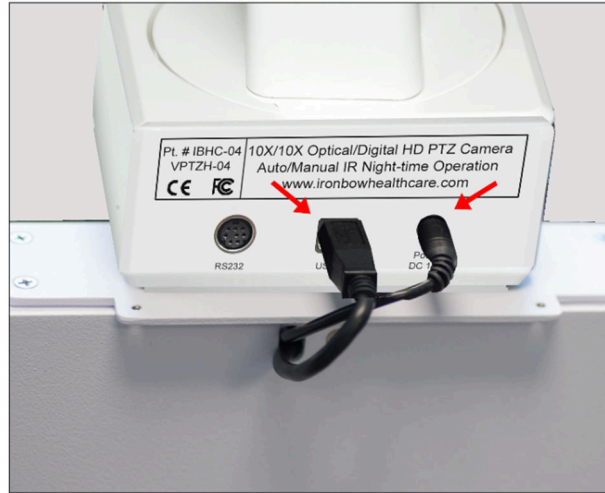
Figure 5 - Connecting the two camera cables
